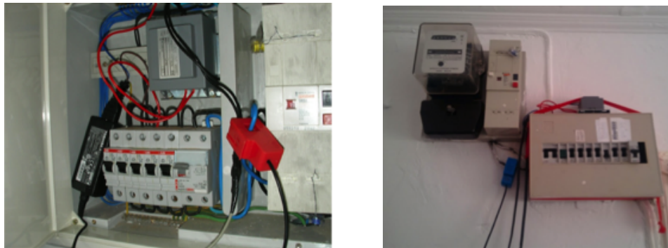
Figure 5: Current and voltage sensors installed in the main power feed
