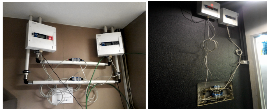
Figure 5. The cold and hot water monitoring systems deployed in two of the three monitored kitchens.
