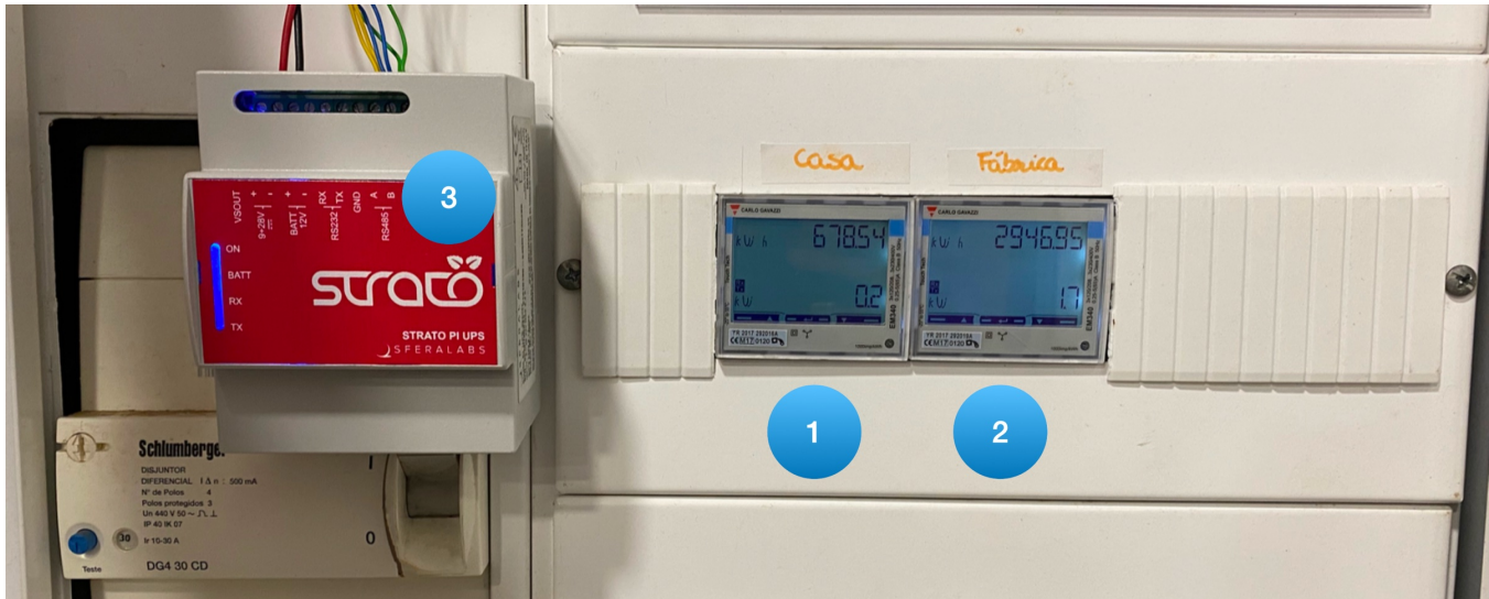
Figure 1: Smart metering infrastructure installed in the main breaker box of one of the participants in the study. Smart matter for household demand (1), smart meter for the factory demand (2), and the strato-pi for data processing and communication (3).
